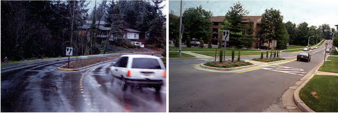
Center planted medians encourage drivers to slow down. Breaks in highway provide safer crossings for pedestrians.
