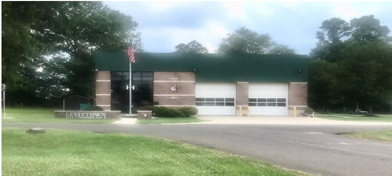
STATION 13 6 County Way Levittown, PA 19055 Owner Levittown Fire Co. #2 Year Built/Renovator 1999
